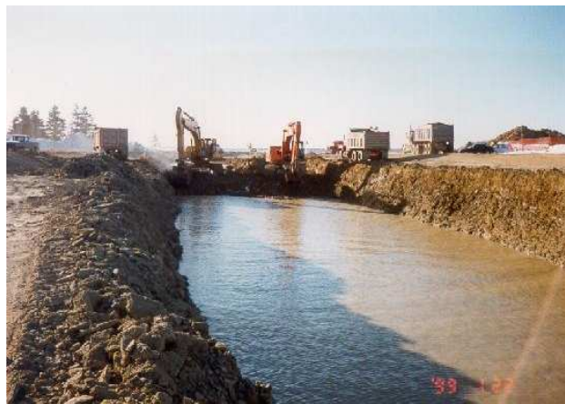
Fig. 12: Final stages of excavation through Whalen Property peninsula.
