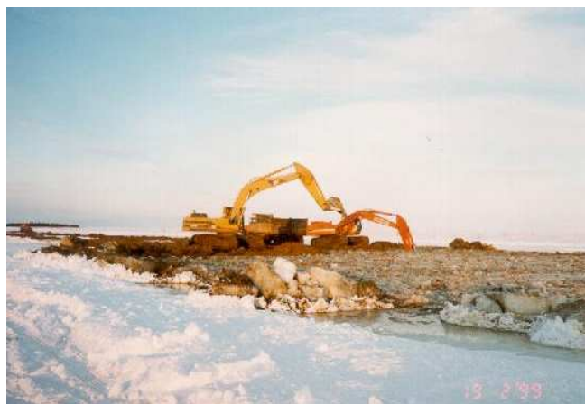
Fig. 7: “Dredging” using on-ice excavators.
