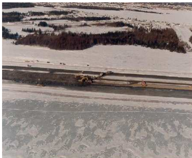
Fig. 10: Aerial picture (west) of channel excavation through McLaughlin Lagoon
