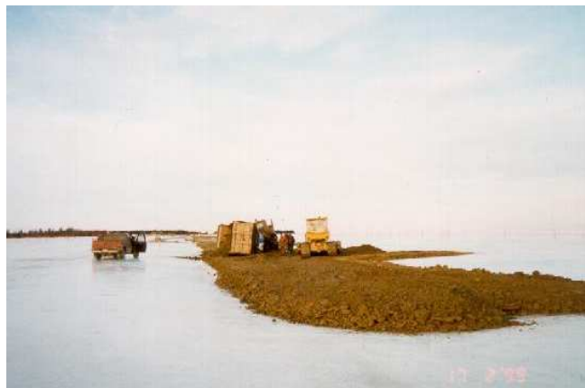
Fig. 6: Placement of excavated soil for temporary on-ice road. Note truck to one side directly on the ice.
