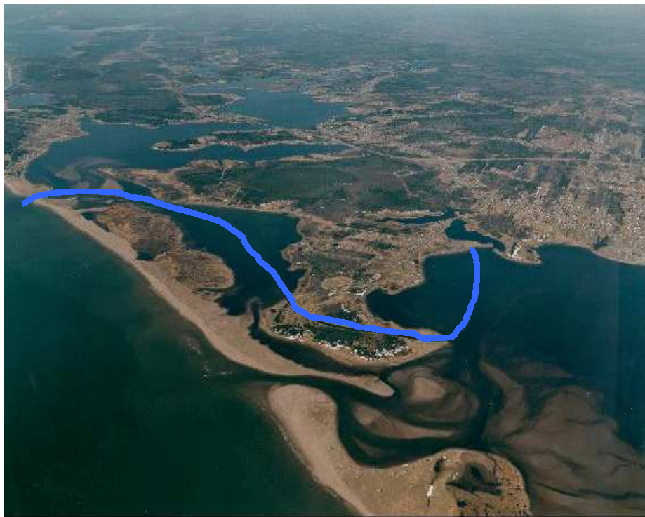
Fig. 14: Aerial view (to the southeast) of the completed channel project
