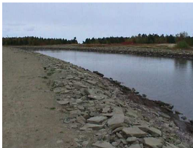
Fig. 13: View of completed channel (Whalen Property section) August 1999. Note shoreline armouring to reduce erosion from shipwake.
